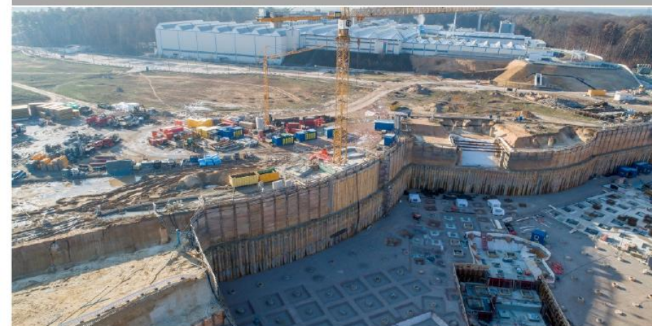
Excavation transfer building & CBM cave
