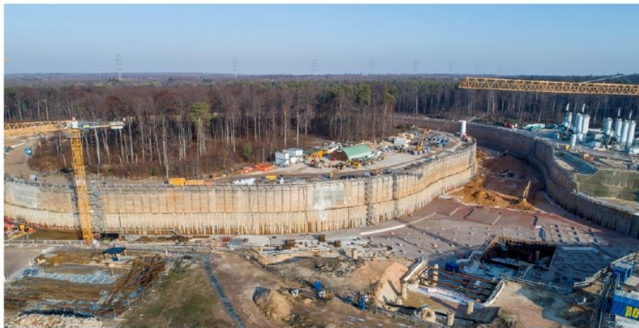
Excavation SIS100 tunnel
